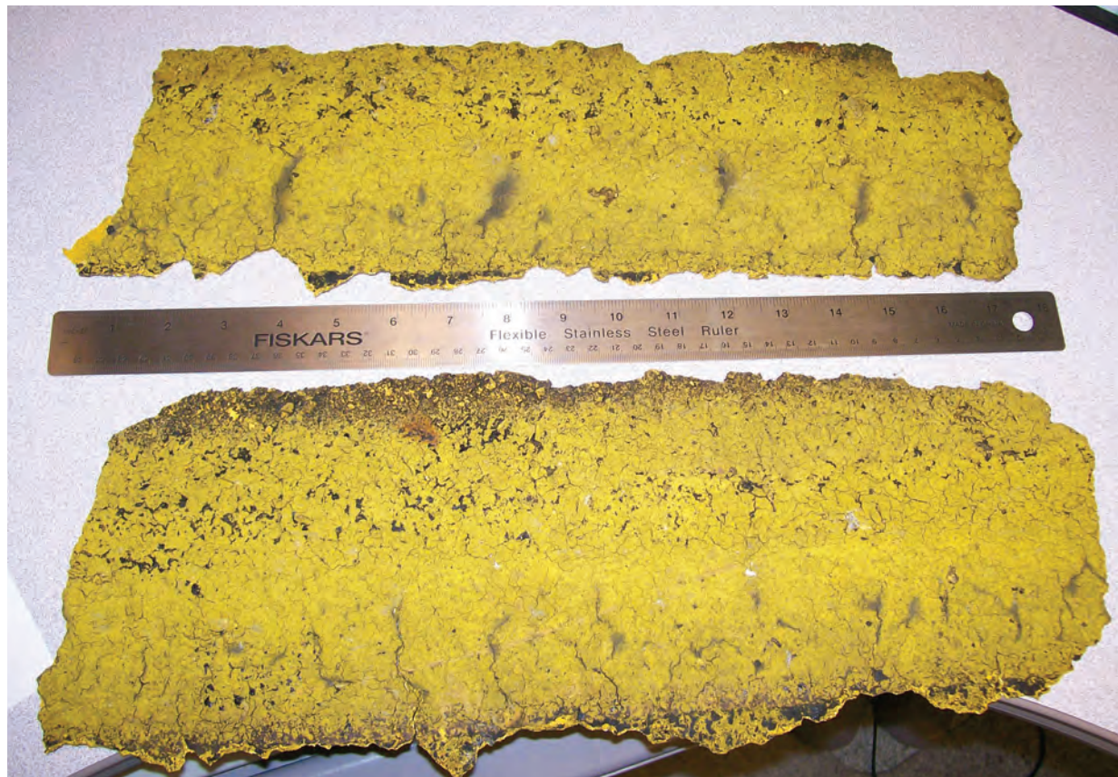
Example of extreme paint chips and FOD if the airside paint is not properly maintained
