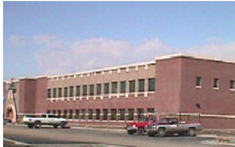
The armory under construction.
