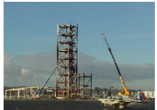
The Paine Field ATCT under construction.
