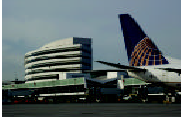
Sea-Tac's New Concourse A
